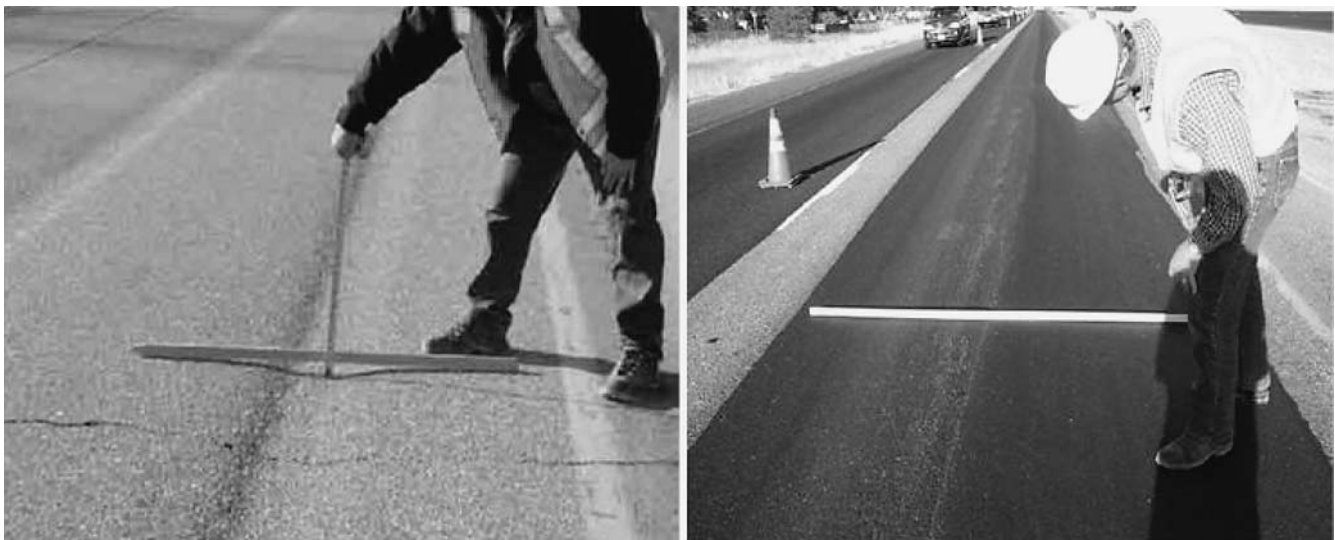
FIGURE 21 Microsurfacing applied to rutting caused by studded tires in Washington State: before and after (Washington State DOT 2009).
